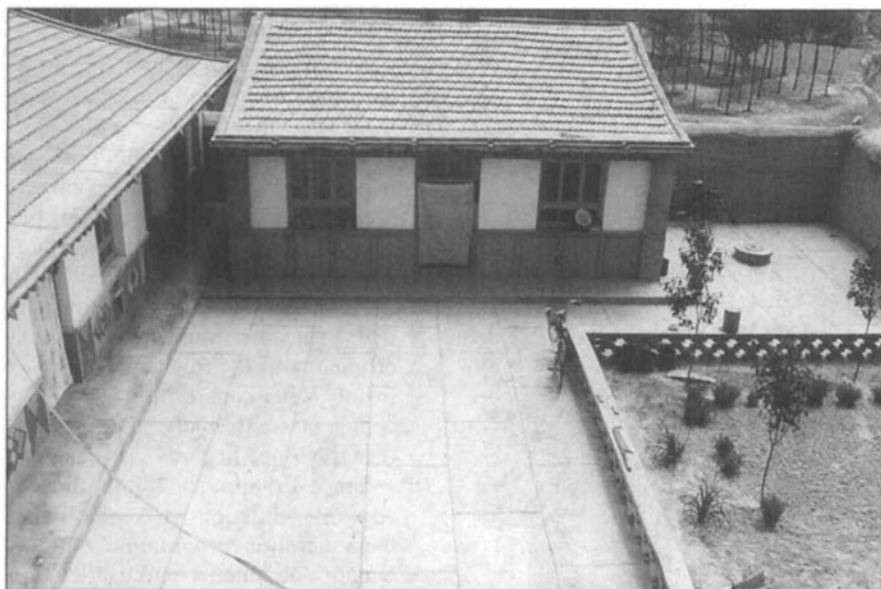
A typical Gansu rainwater catchment — a tiled roof and concrete-lined courtyard for rainfall collection, and an underground tank with a capacity of 15 to 20m 3 .
