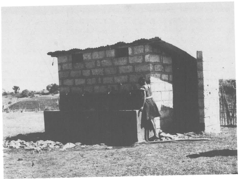
Process: Fetching water from a Comfort Station — a combined public standpost and sanitary facility.
