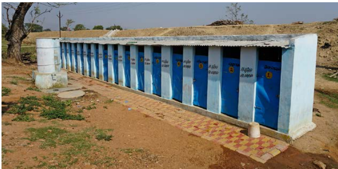
Villagers in Goba -Ganjam district- who do not have space for a toilet in the home, have a personal latrine with a lock on the community ground
