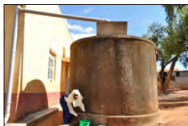
WaterAid supported the construction of the rain harvesting water tank that provides safe water to schools girls for cleaning themselves.
