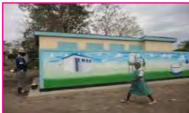
After the intervention
