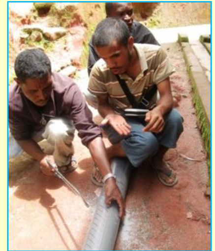
Masons cut slots in casing in Madagascar
