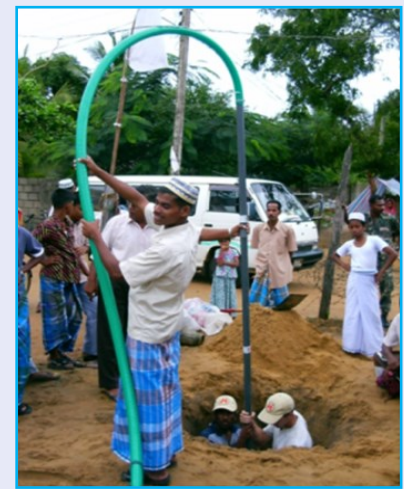
Sludging technology being used in Kenya
