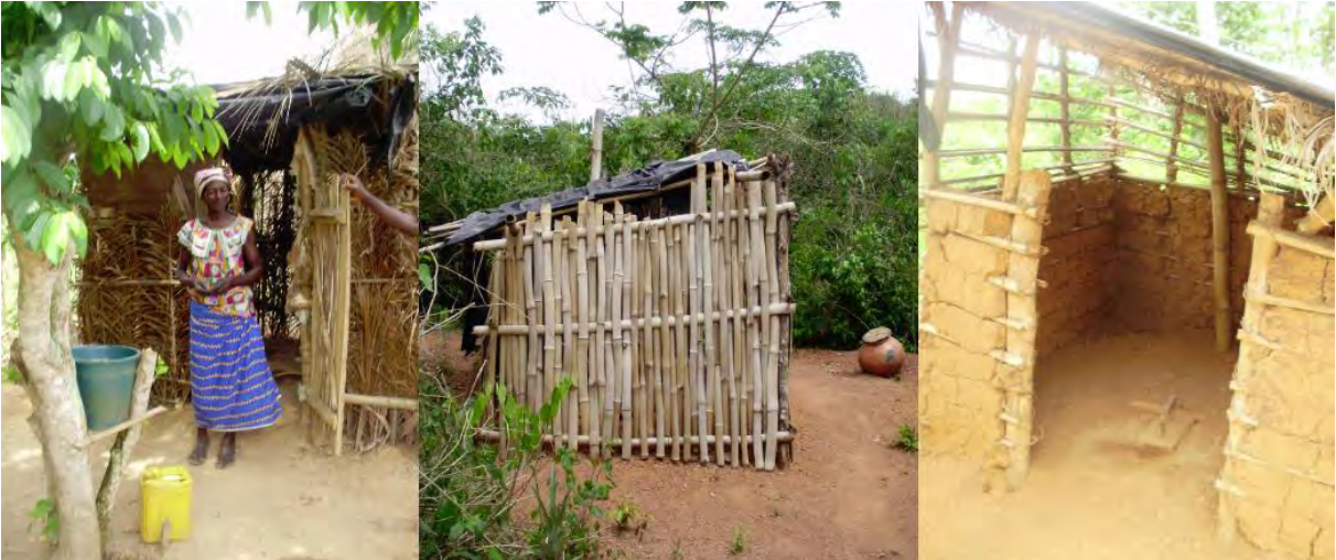
Figure 32: latrines constructed by members of the Koliete community, Ghana.
