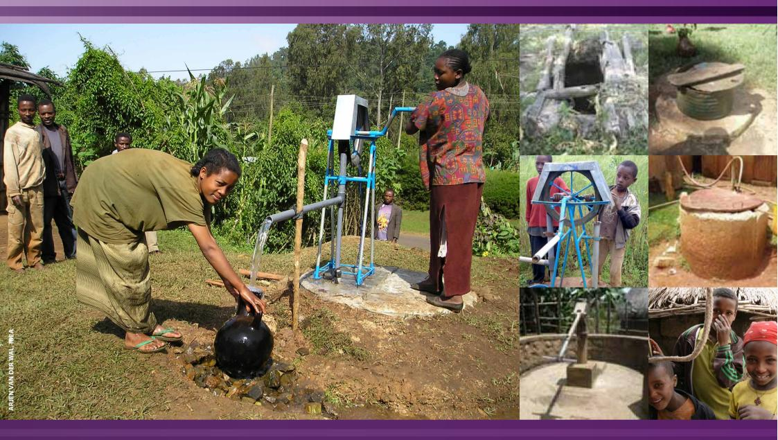
Family wells can provide safe water, but often do not. Wells with simple protection to stop water running into the well, or a rope pump, are 3-5 times more likely to provide safe water than unprotected wells.
