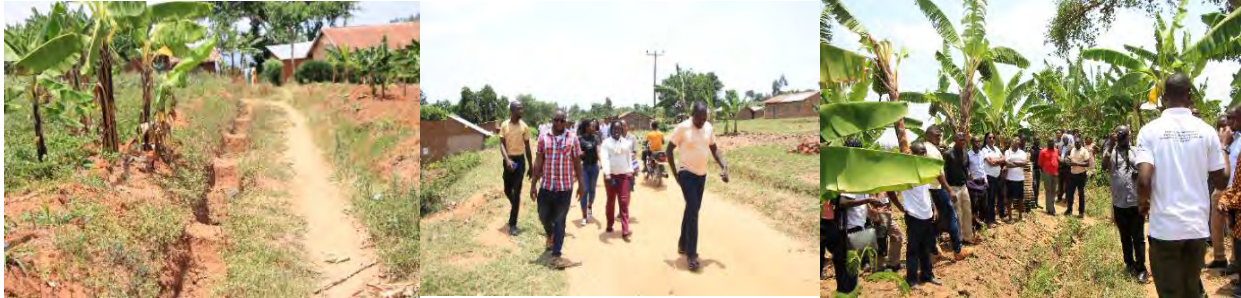
Figure 7: A team visit flood control structure at farm pot Bukutu in Manafwa district
